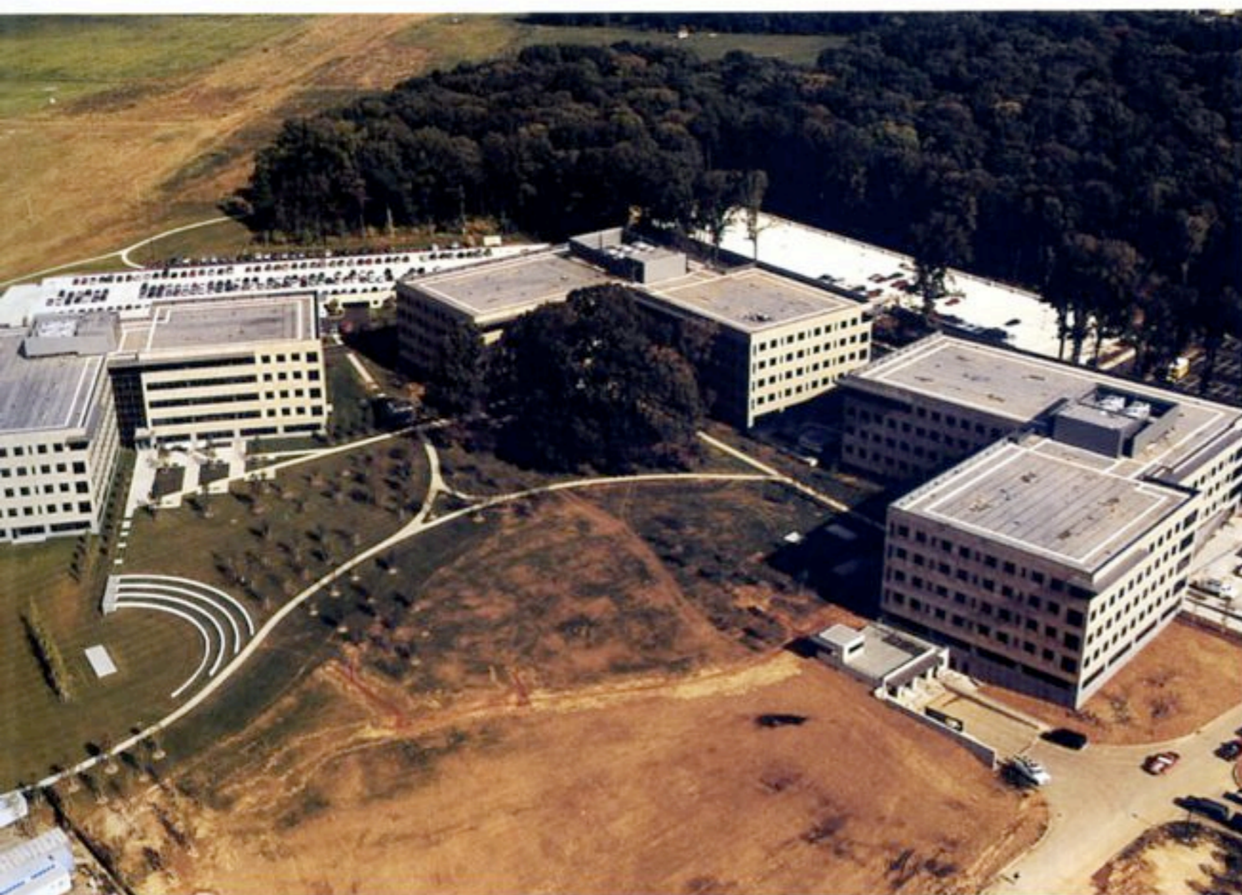
Aerial view of the Plainsboro site. Buildings One, Two, and Three are shown from left to right.
